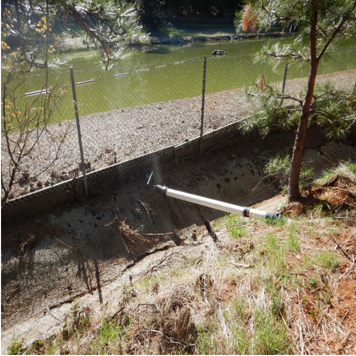
Photo No. 9: Piping from tailwater collection ditch to the wastewater pond.
