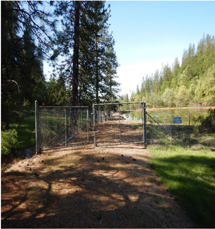
Photo No. 1: Security fence with locking gate surrounding the wastewater pond.
